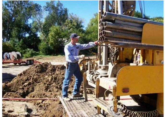
John Warrick drilling a 2-Ton GeoExchange system for Habitat for Humanity
